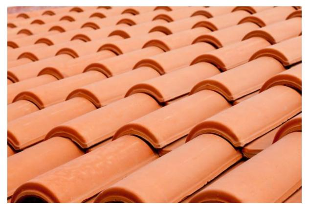
Terracotta is naturally orange in color due to the oxidation of iron that occurs when the product is exposed to high temperatures. Image source: Shutterstock user Pi-Lens
