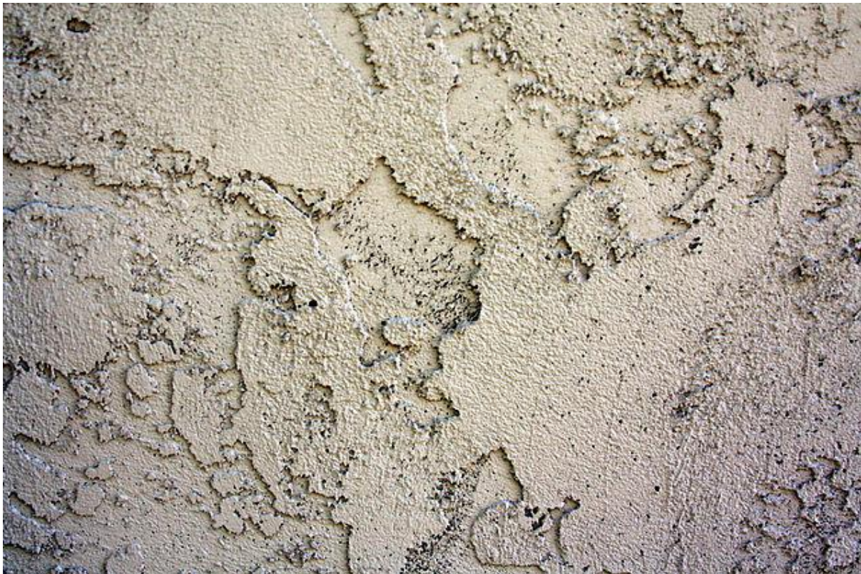
The texture of stucco can alter the overall color appearance. Image Source: Wikimedia user Dante Alighieri
